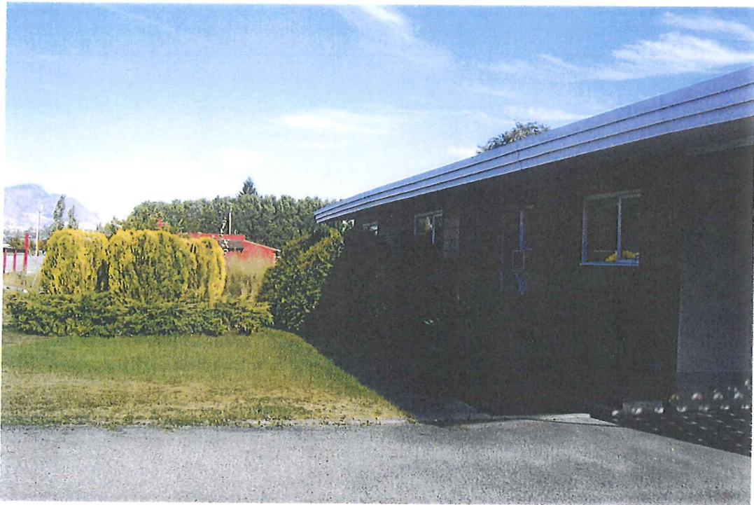
EXISTING HOUSE FRONT YARD (ON KLO)
